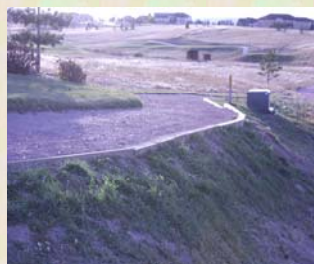
Rebuild trail with retaining wall
